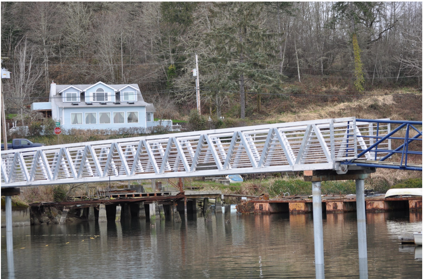
LIC Wharf after construction, February 12, 2011
