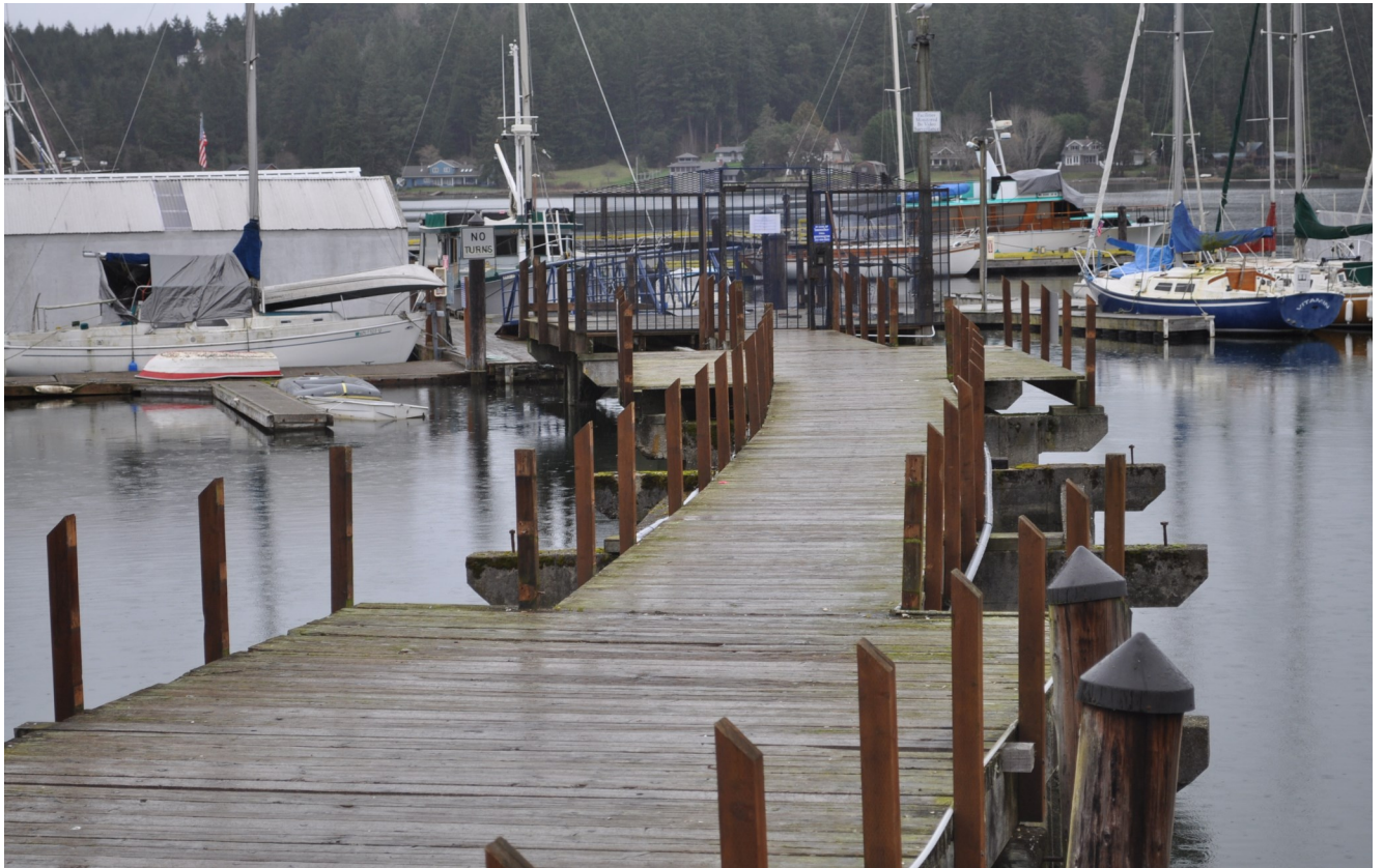
LIC Wharf ready for demolition, January 18, 2011.
