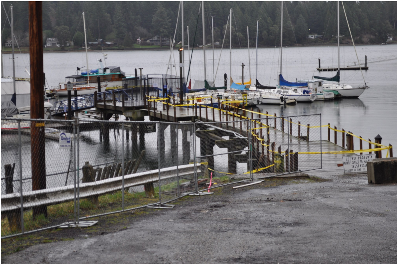
The wharf, after the work party and after security fence installed
