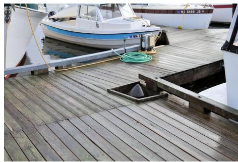
Look at the Piling
