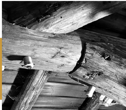
Custom-cut under purlins, beams, and struts, complete with 1930's porcelain knob insulators, part of the original wiring system (no longer in use, obviously).
